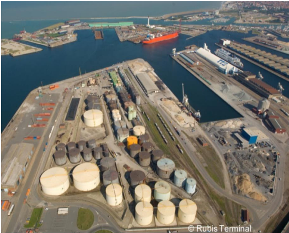
Figure 63: Rubis Terminal installations on wharf n°5, port of Dunkirk
