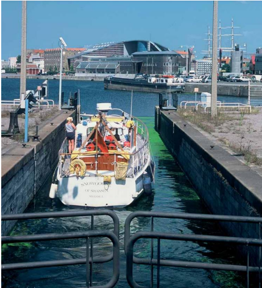
Figure 66: The Darse n°1 lock, view towards the port
