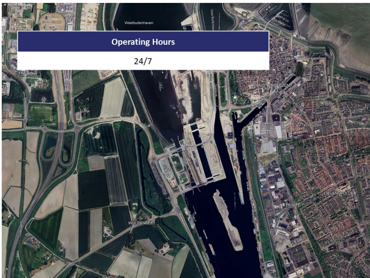
Figure 48: Terneuzen lock complex
