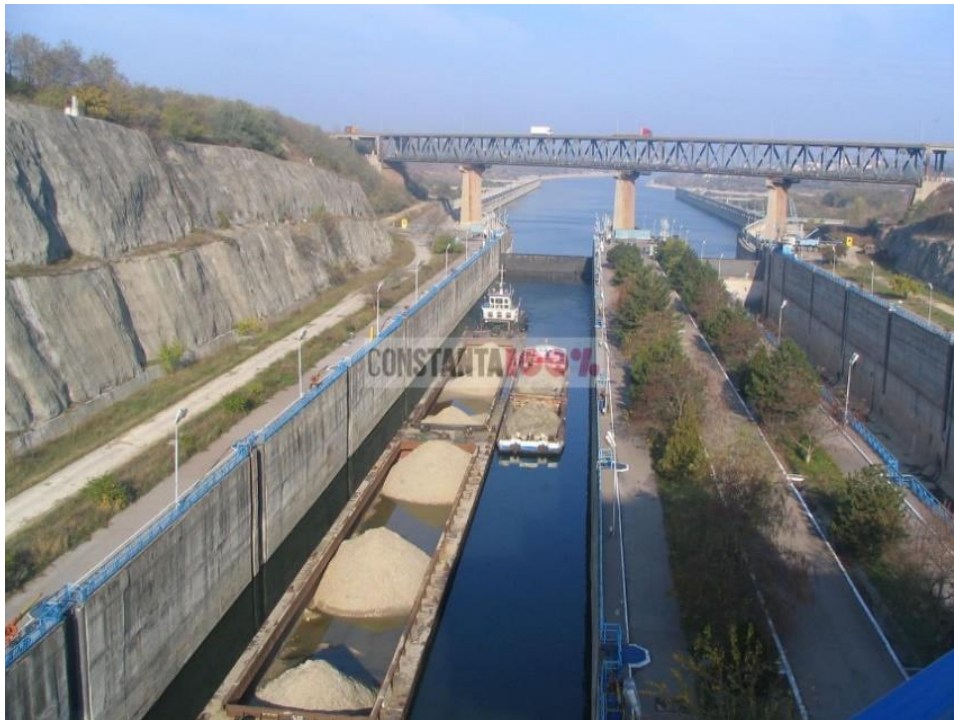
Figure 133. Černavoda lock chambers
